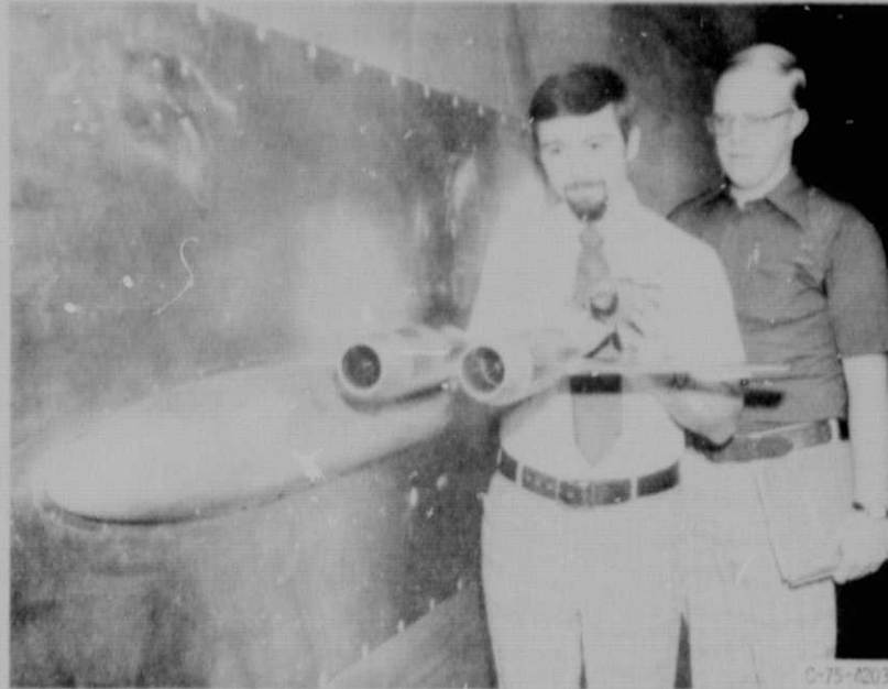
Figure 1. - U. S. B. propulsion integration model in wind tunnel.
