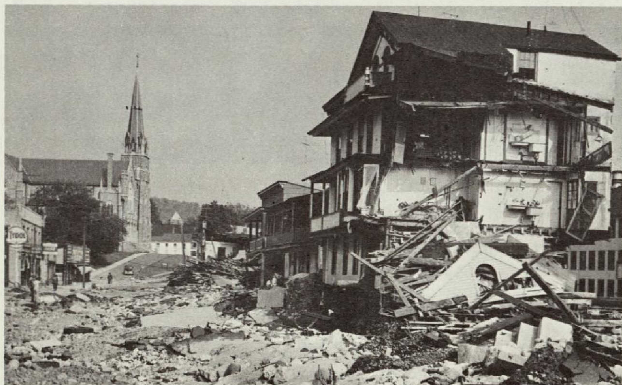
AUGUST 1955 FLOOD DAMAGE AT WINSTED, CONNECTICUT
