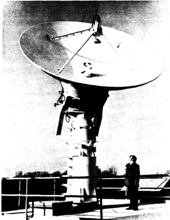
Figure VII-11. - 5-Meter SHF Cassegrain Antenna.
