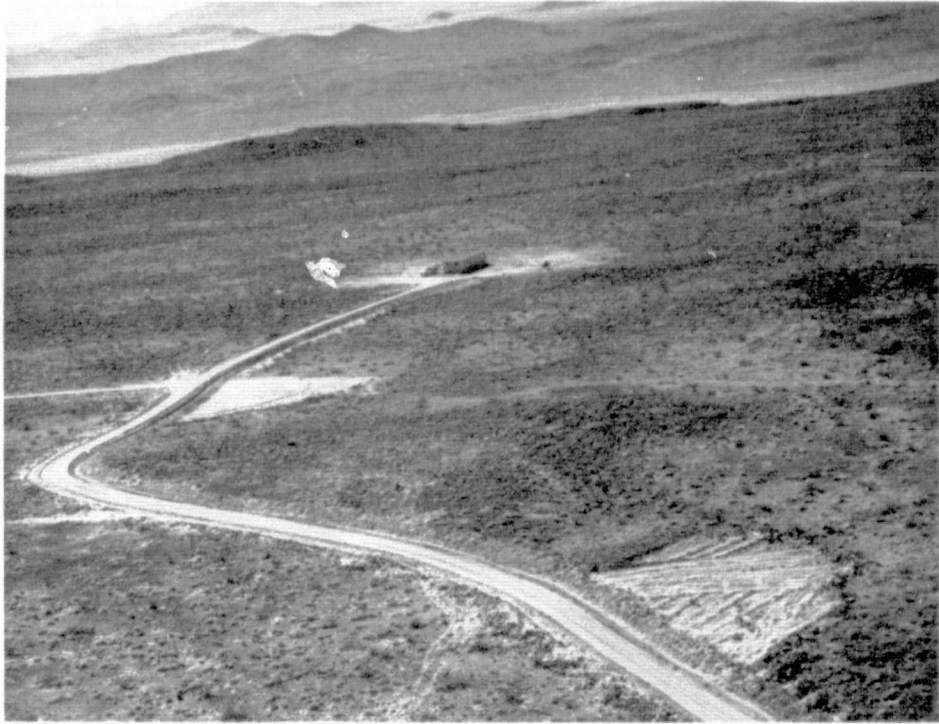
Fig. 41. OSR access road
