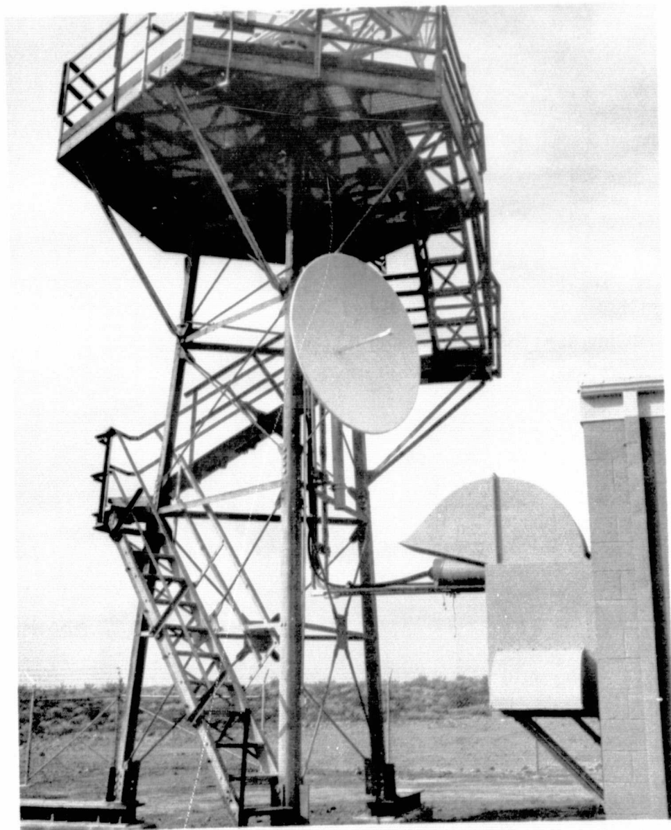
Fig. 37. Radar site microwave antenna
