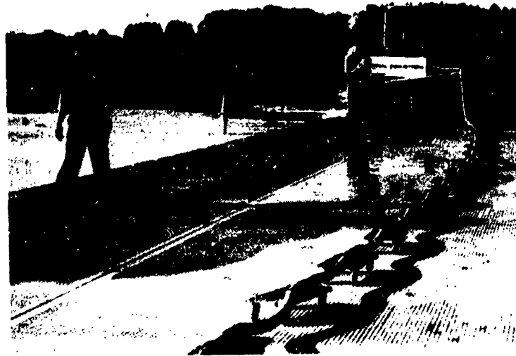
Figure 5.- Space shuttle landing facility at KSC with pavement grooving machine (diamond blades).
