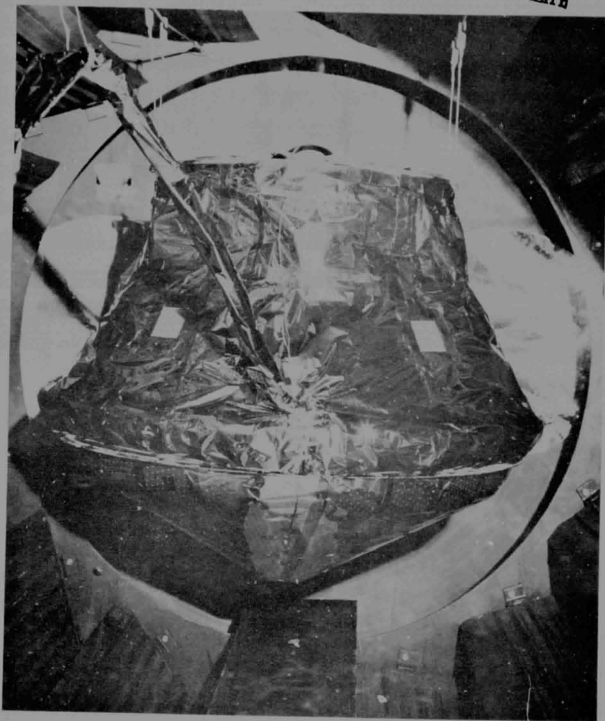
ADAPTER INSTALLATION IN TEST CHAMBER
