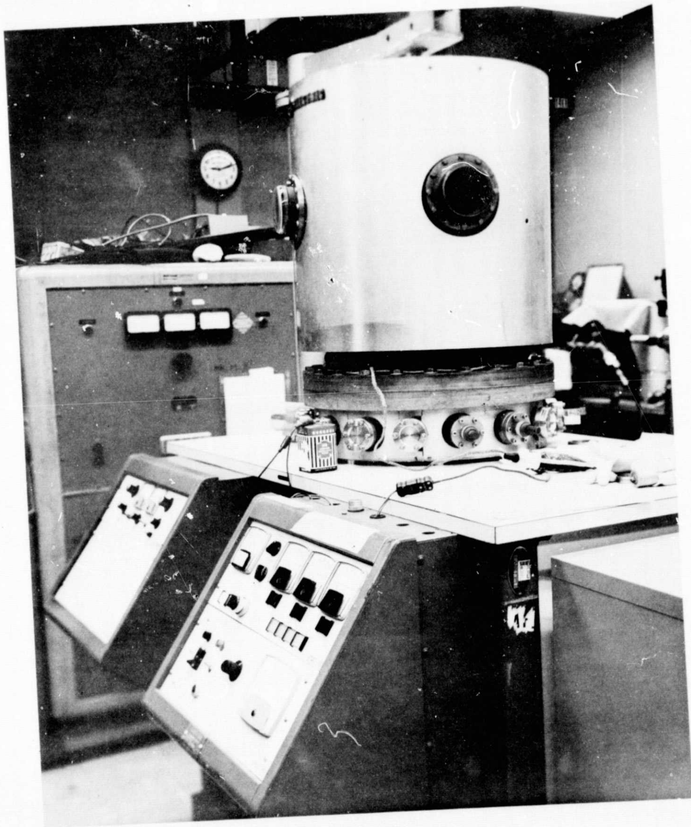
Figure 1. Basic GE Triode Pumped Vacuum Facility, 1200 \ell/s
