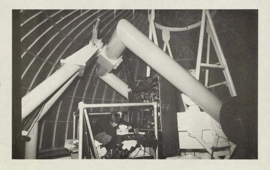
Figure 4. The laser box attached to the declination cable of the telescope.
