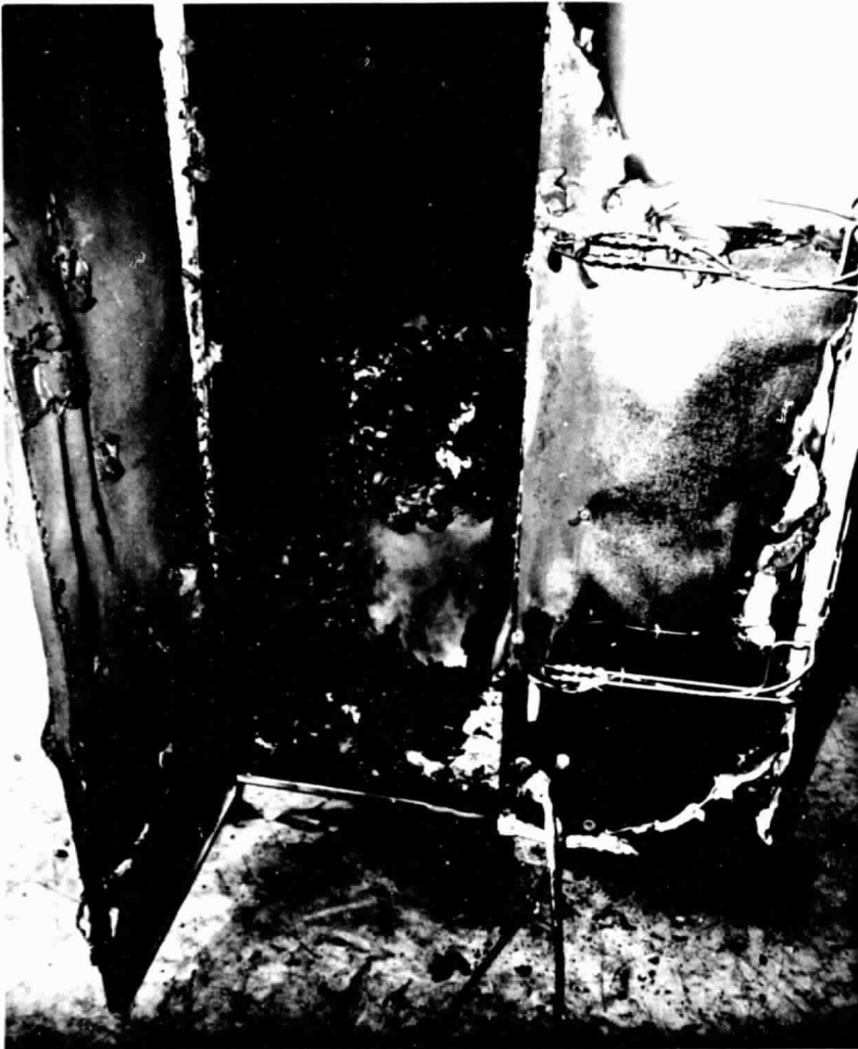
RESIDUAL FUEL REMAINING
