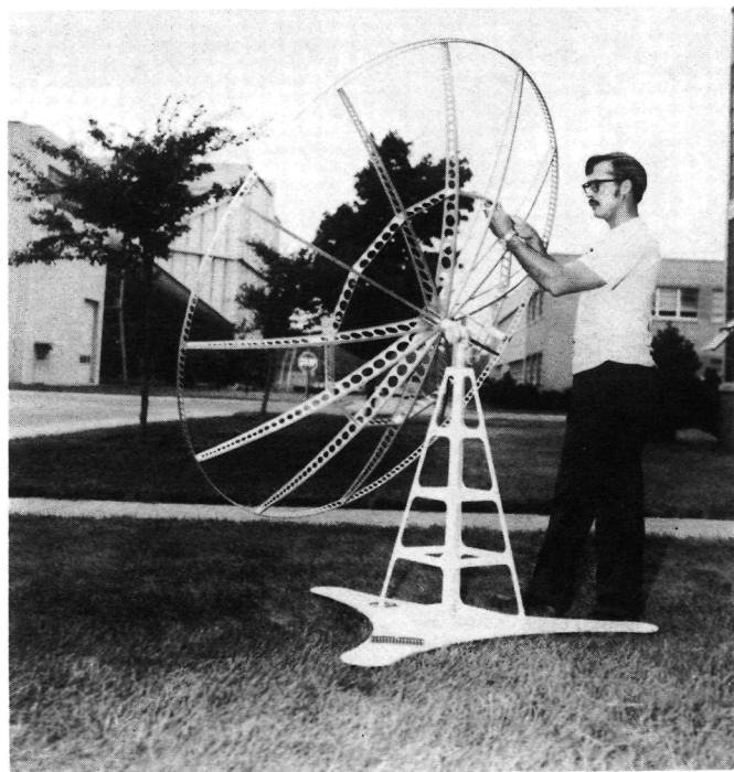
Figure 14. - Concentrator support structure.
