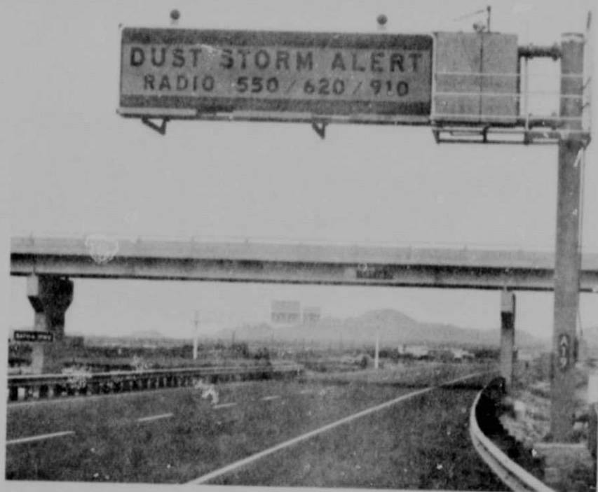
Photovoltaic powered dust storm warning sign on Interstate 10 between Phoenix and Tucson.
