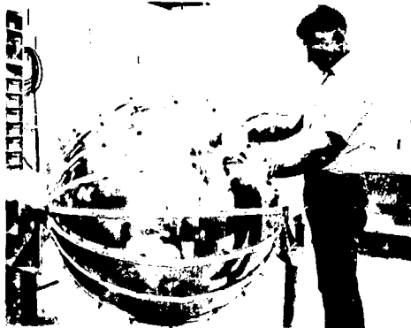
(B) FAB SPRING ASSEMBLIES, BOND TO TANK. COMPRESS WITH KEVLAR STRANDS.
