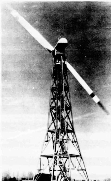
Figure 1. Mod-0 Wind Turbine - Original Configuration with Stairs and Rails.
