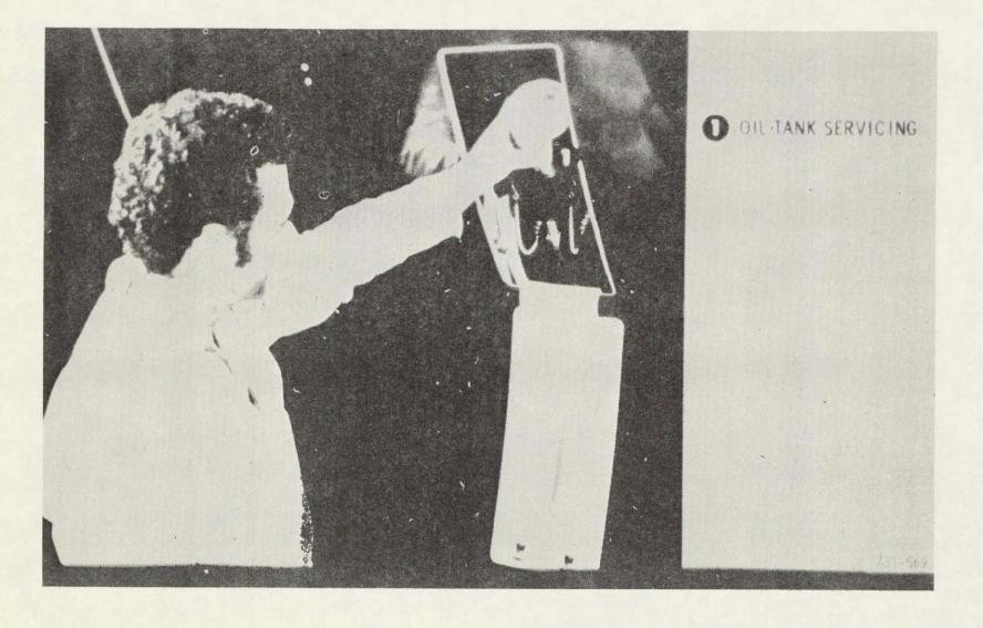
Figure VII-1. CF6 Nacelle, Accessibility, Oil Tank Servicing.
