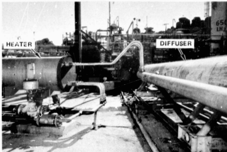
Figure 84. Altitude System Diffuser and Ejector Gas Heater
