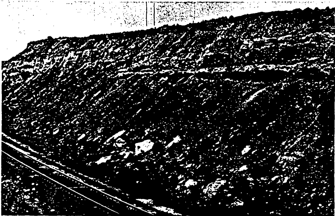
Figure 7.10. The Chicago, St. Paul, Milwaukee and Pacific Railroad cut through the pendant bar at the downstream end of the Marengo loess hill.
