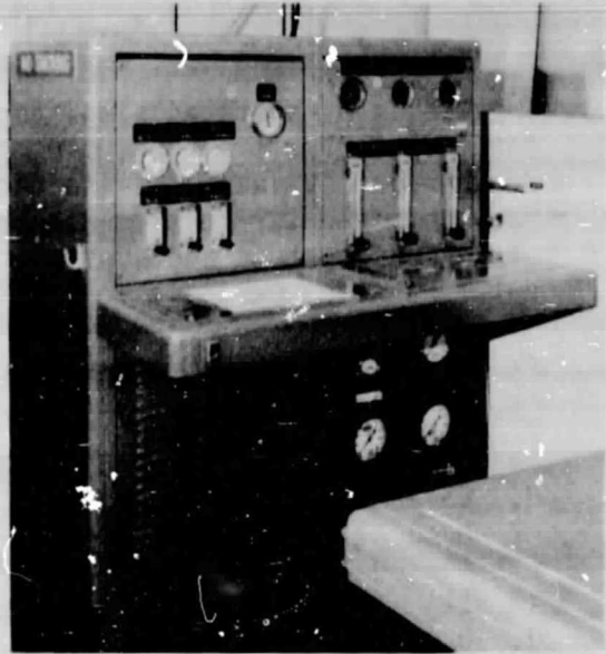
Figure 4.- Environmental control and liquid cooled garment system console.
