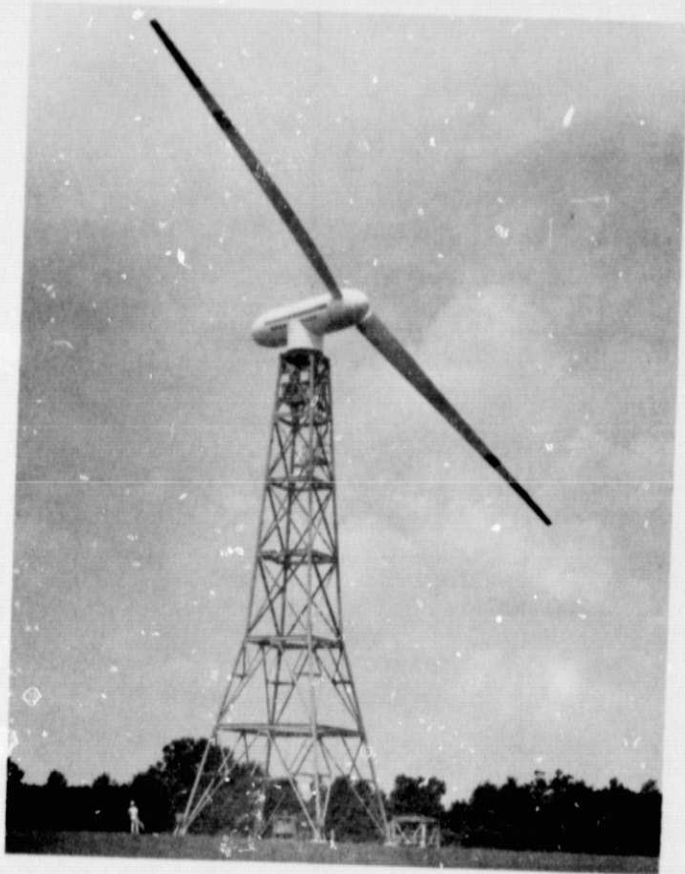
Figure 1. - 100 KW Wind Turbine.
