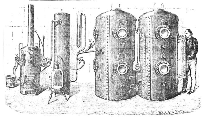
3. The beginnings of aeronautic medicine. Bert's pressure chamber constructed in 1869, consists of two chambers connected by an air tight door. On the left is a vacuum pump (operated by steam) and a manometer. With the aid of this pressure chamber, Bert was able to study the effects of oxygen defficiency on man.
