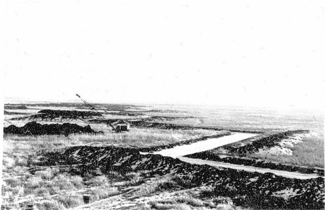
Figure 5. Photograph illustrating level ditch construction.
