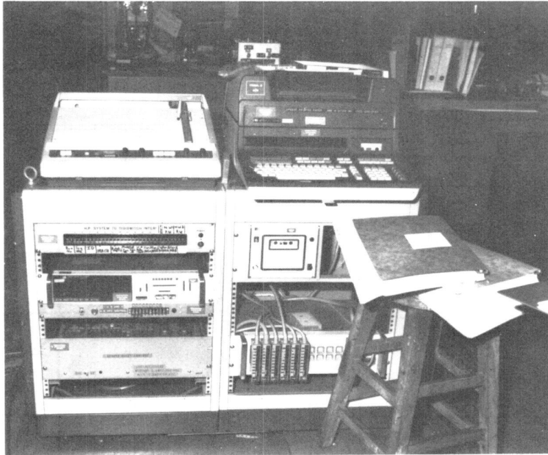
Figure 13.— Calculator console for dynamic data control.
