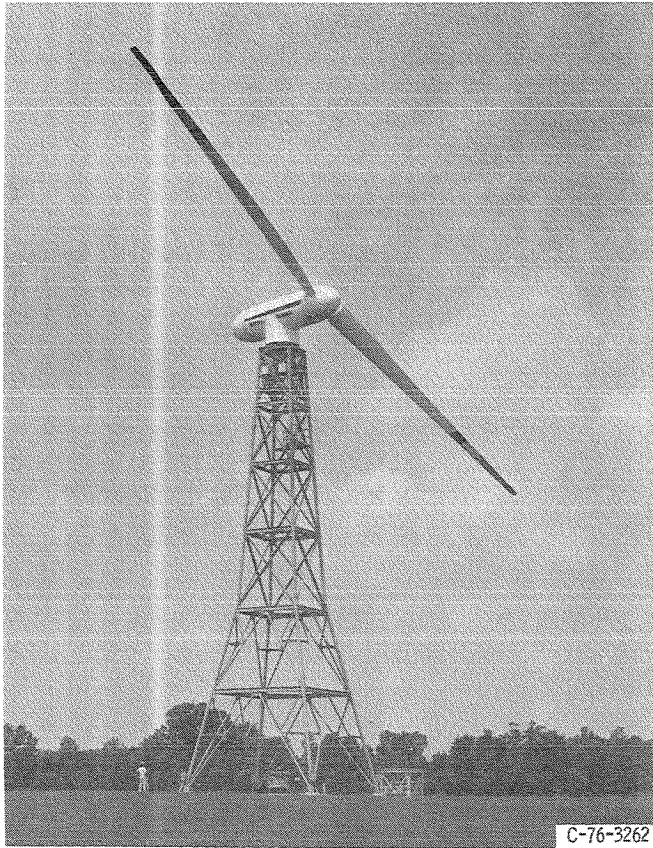
Figure 1. - Mod - 0 wind turbine before installation of softening fixture.
