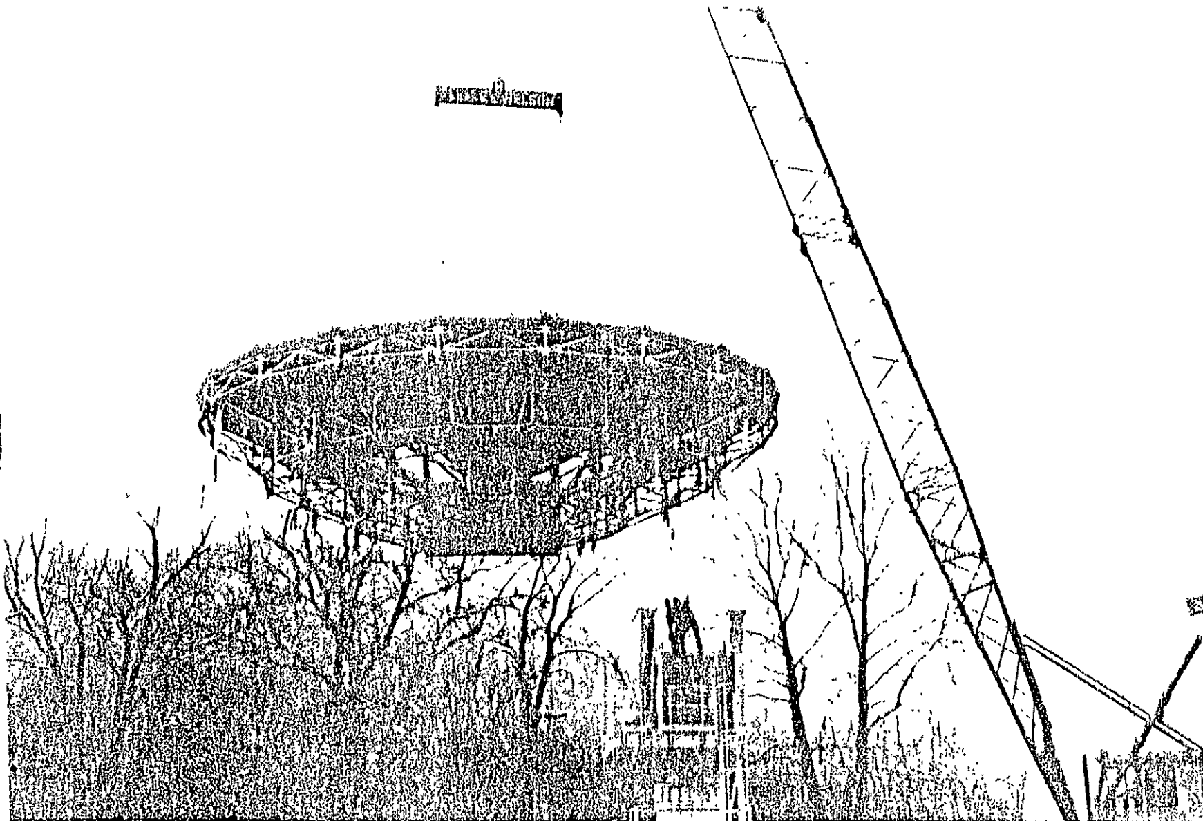
FIGURE 67. TYPICAL REFLECTOR STRUCTURE/PANEL ASSEMBLY BEING LIFTED
