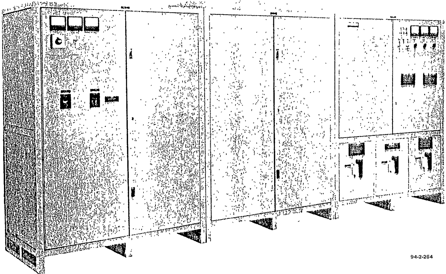
FIGURE 17. INTERNATIONAL POWER MACHINES 330 KW CONVERTER AND INVERTER ASSEMBLED IN UPS CONFIGURATION
