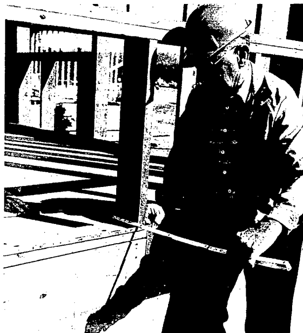
Figure 17.- Wall structure showing 2- by 6-in. studs.
