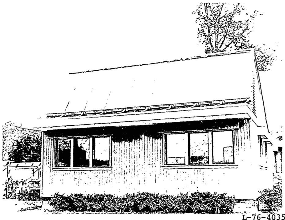
Figure 3.- Tech House solar panels.
