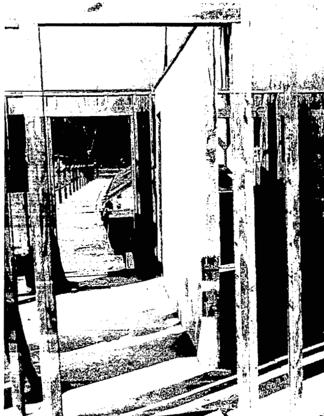
Figure 18.- Reconstituted sawdust studs and precast wall.
