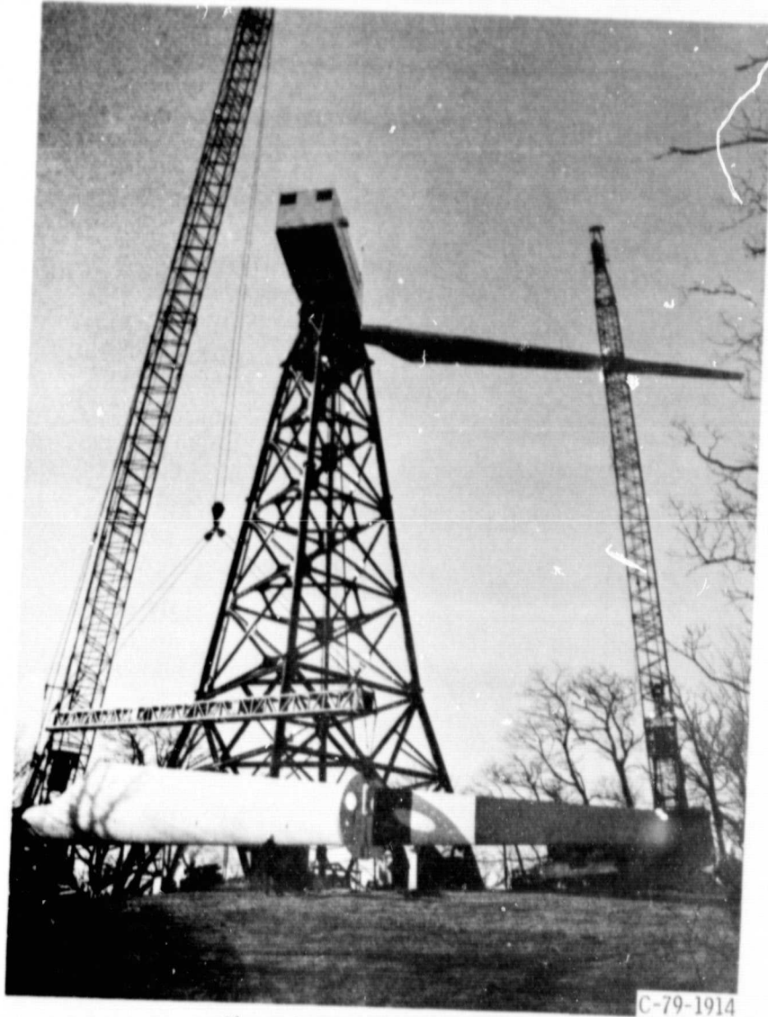
Figure 17. - Blade installation.
