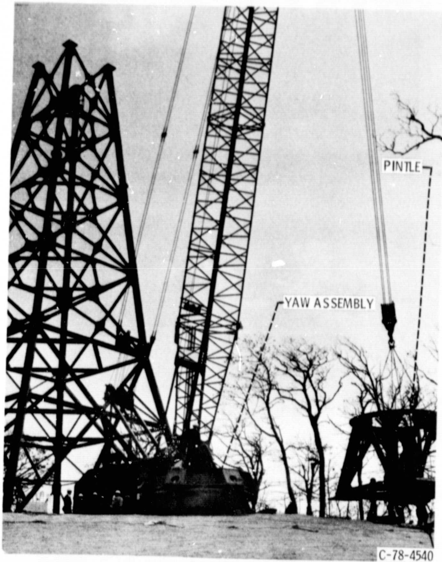
Figure 13. - Pintle installation.
