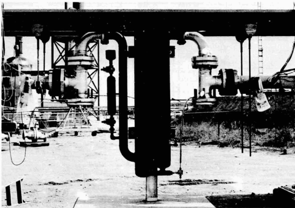
Figure 8-22. Linde Hydraulic Back-Pressure Valve Arrester Test Installation
