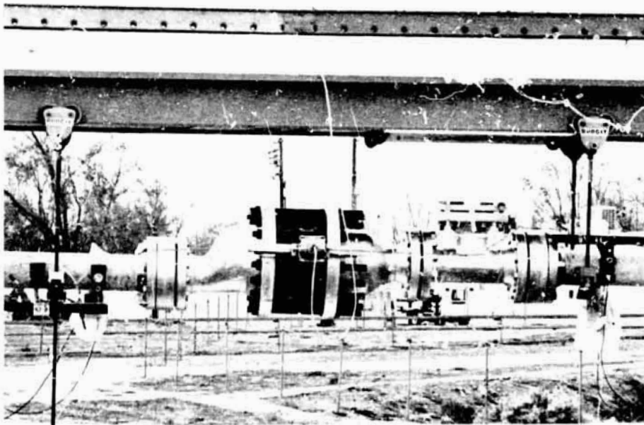
Figure 13-8. Shand and Jurs Spiral-Wound, Crimped Stainless-Steel Ribbon Arrester Test Installation with Direct Connect Inlet
