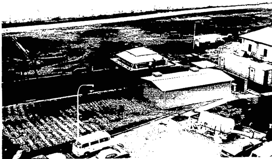
Fig. 1. Energy Storage Boiler Tank at the Naval Research Laboratory
