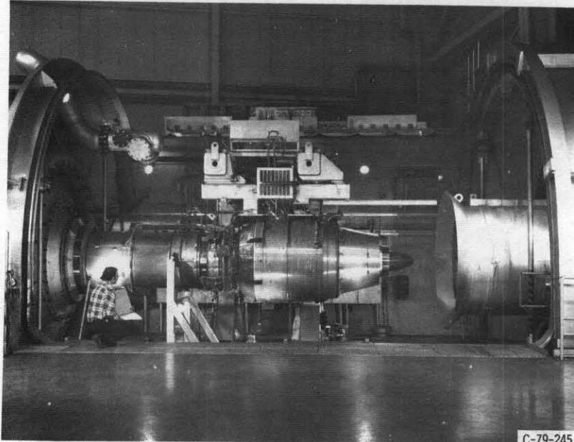
Figure 5. - Single stage fan, turbfan engine installation.
