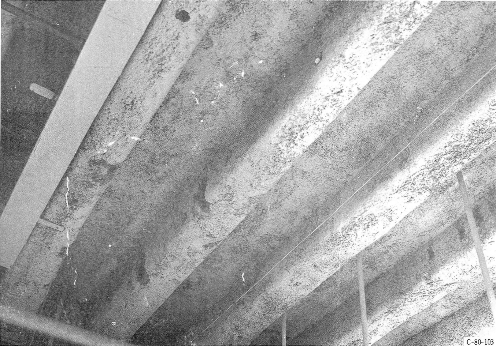
Figure 1. - Spray-applied ceiling insulation.
