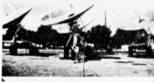
FIG. 4. QUADRANT TEST SOLAR COLLECTORS
