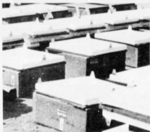
FIGURE 2. MIRROR FACETS WITH FLEXURE ATTACHMENT HARDWARE
