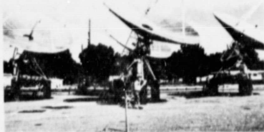
FIG. 4. QUADRANT TEST OF SHENANDOAH SOLAR COLLECTOR
