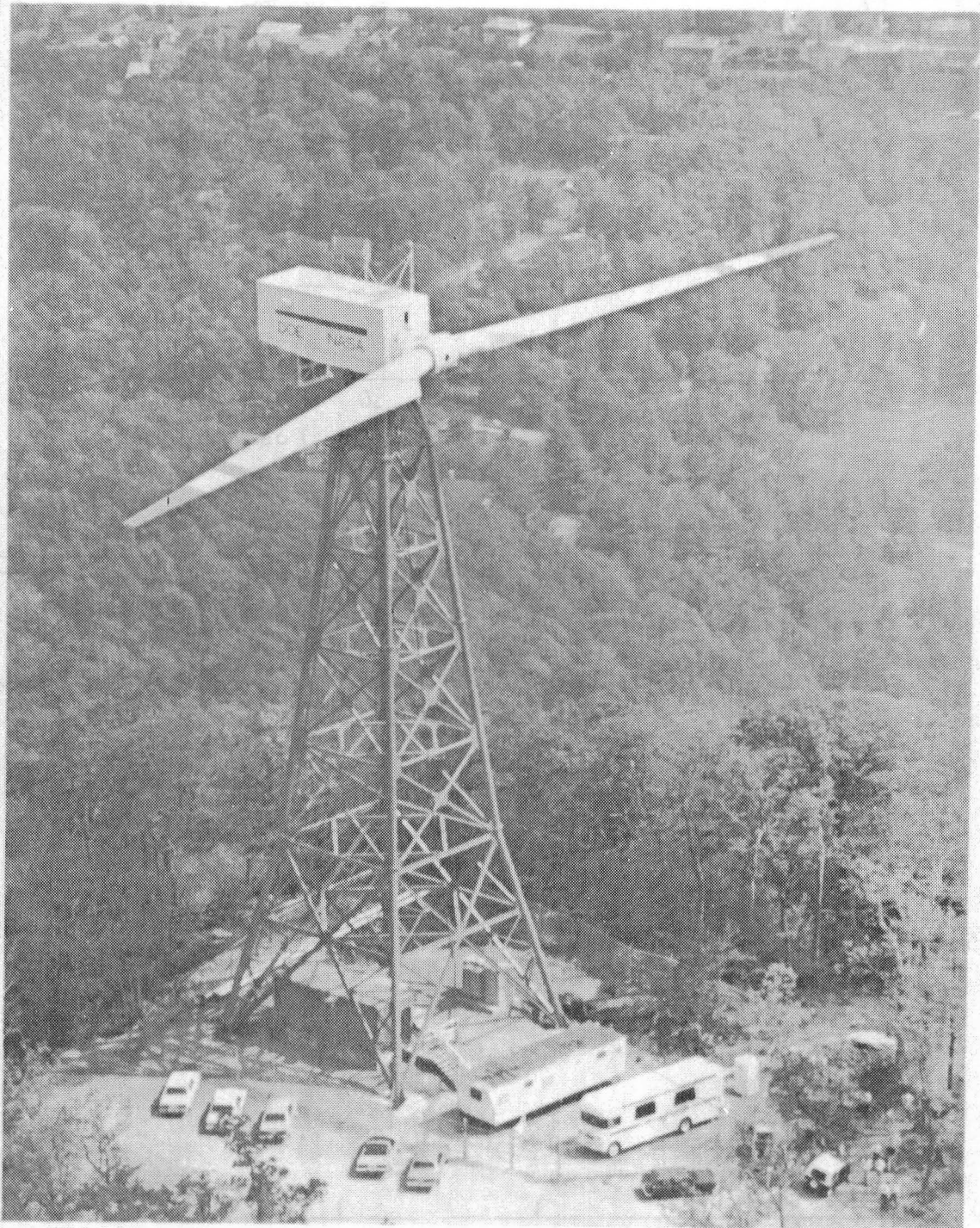
Figure 1.- DOE/NASA 2000 KW Experimental Wind Turbine
