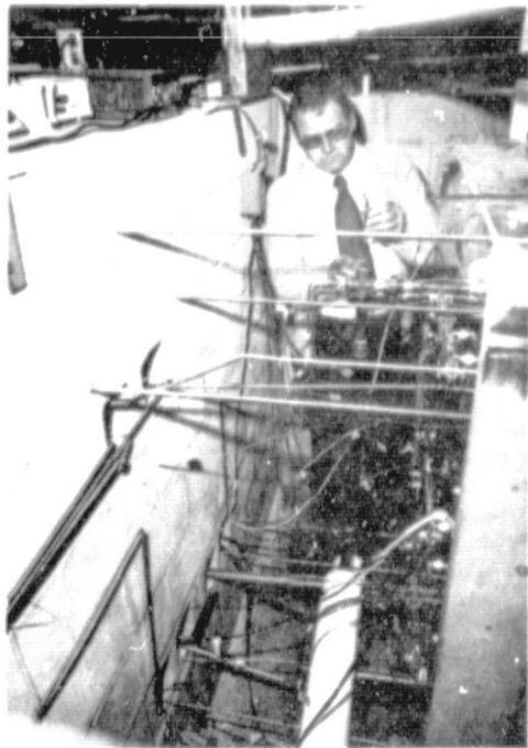
B. Valve Extender Rods, Instrumentation Wires, and Hydraulic and Pneumatic Lines
