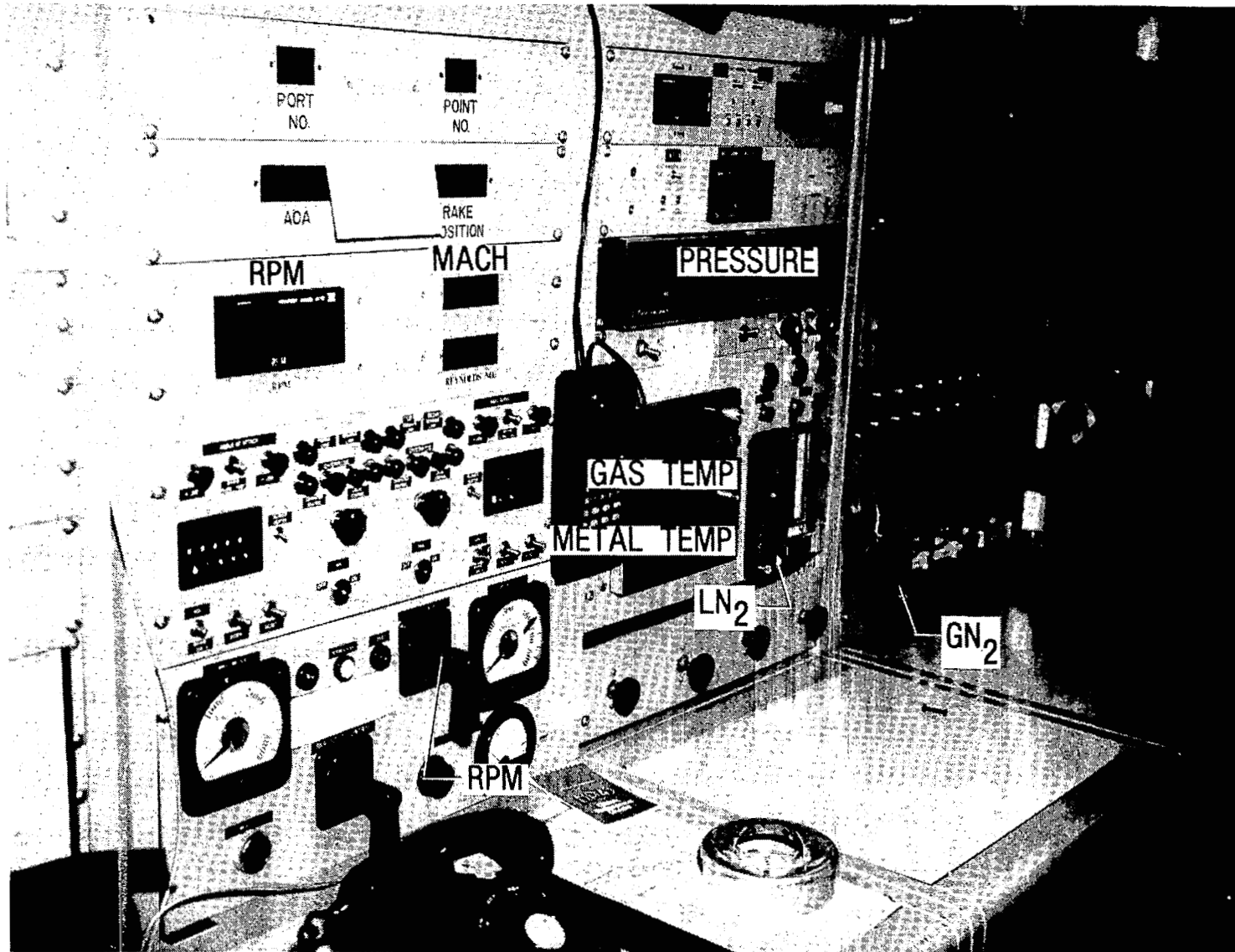
Figure 7.- Control panel 0.3-m TCT.
