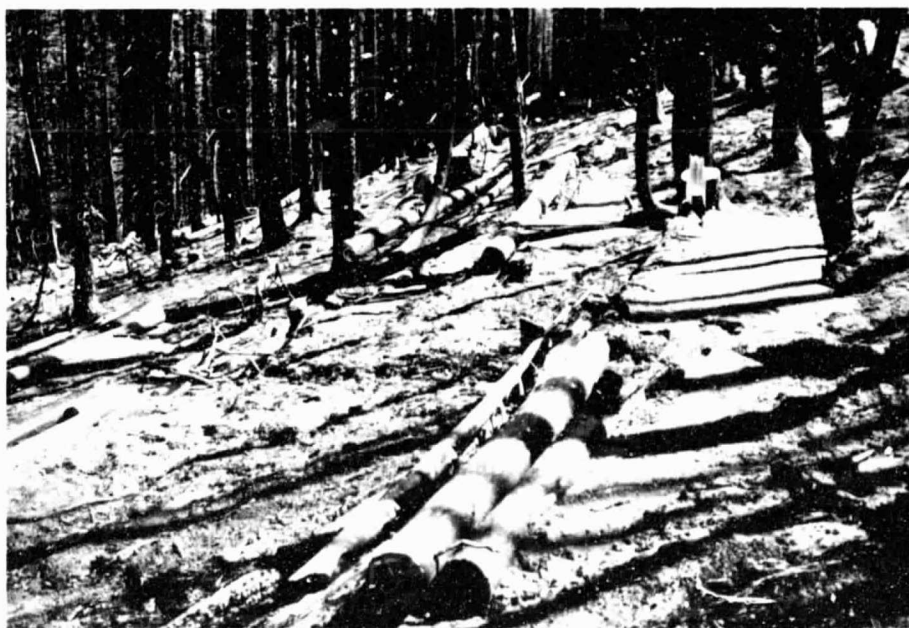
Figure 7B. On long slopes where large volumes of water could be predicted to move overland, snags were felled parallel to contours to break up flow and collect silt deposits.
