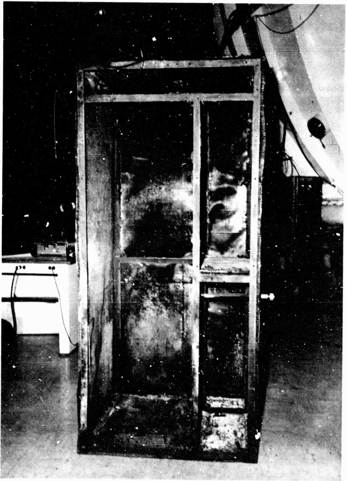
FIGURE 20 MODULE A INTERIOR WITH FRONT WALL AND DOOR REMOVED
