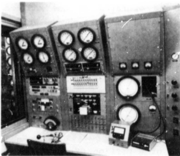
ENGINE TEST CONSOLE
