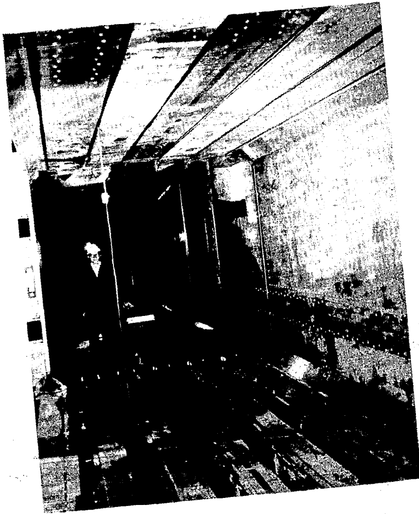
Figure 22.- Slotted-wall test section.
