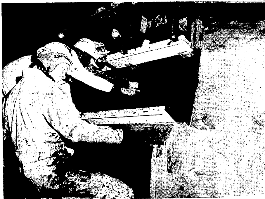
Figure 27.- Installation of internal insulation.
