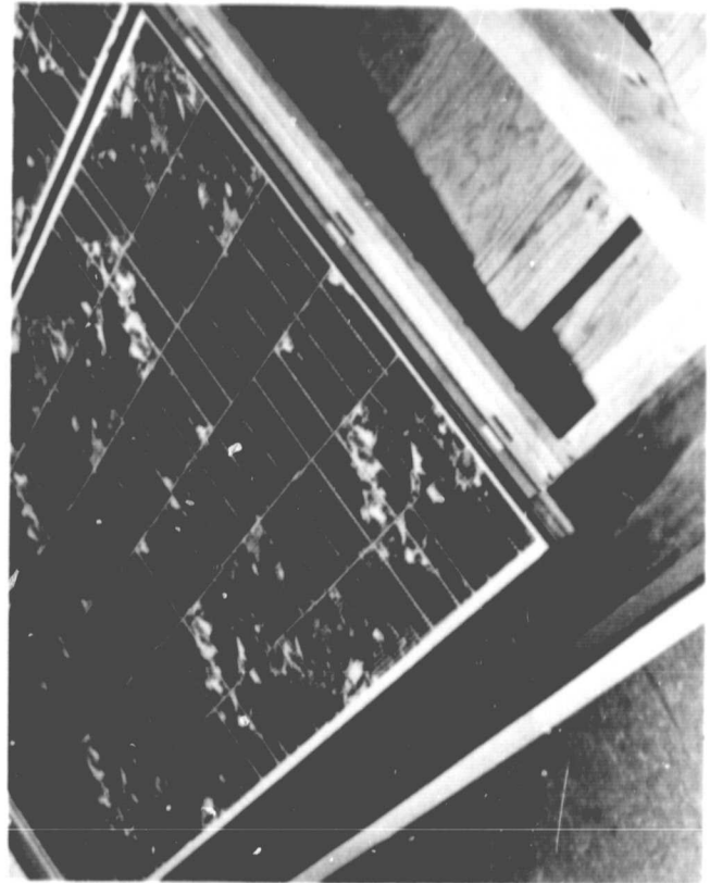
Figure 3-4 c Module Interface with Support Hardware at Eave and Rake
