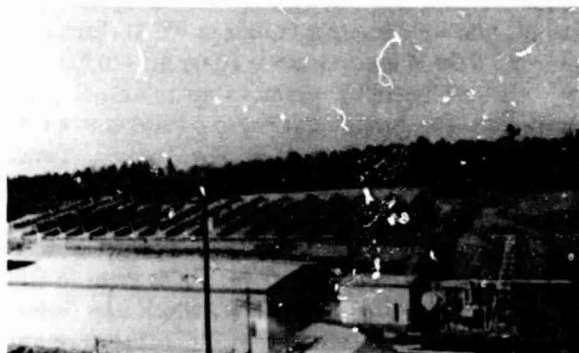
Parabolic Troughs Installed at Dow Chemical Plant in Dalton, Georgia
