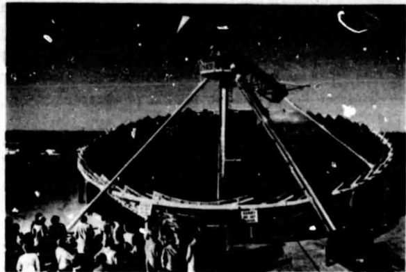
Crosbyton Solar Power Project Using Hemispherical Bowl
