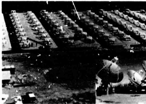
Solar Total-Energy Plant Under Construction in Shenandoah, Georgia, May 1981
