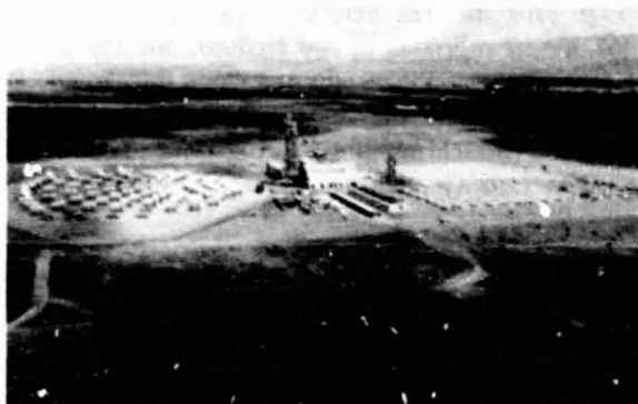
Field of Heliostats and Parabolic Troughs at Small Solar Power System Project in Almeria, Spain
