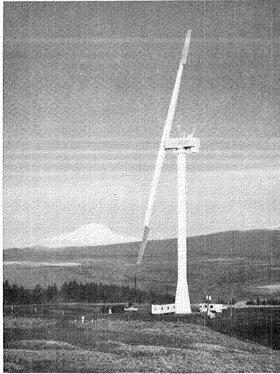
Figure 4. - Mod-2 2500 kW wind turbine.
