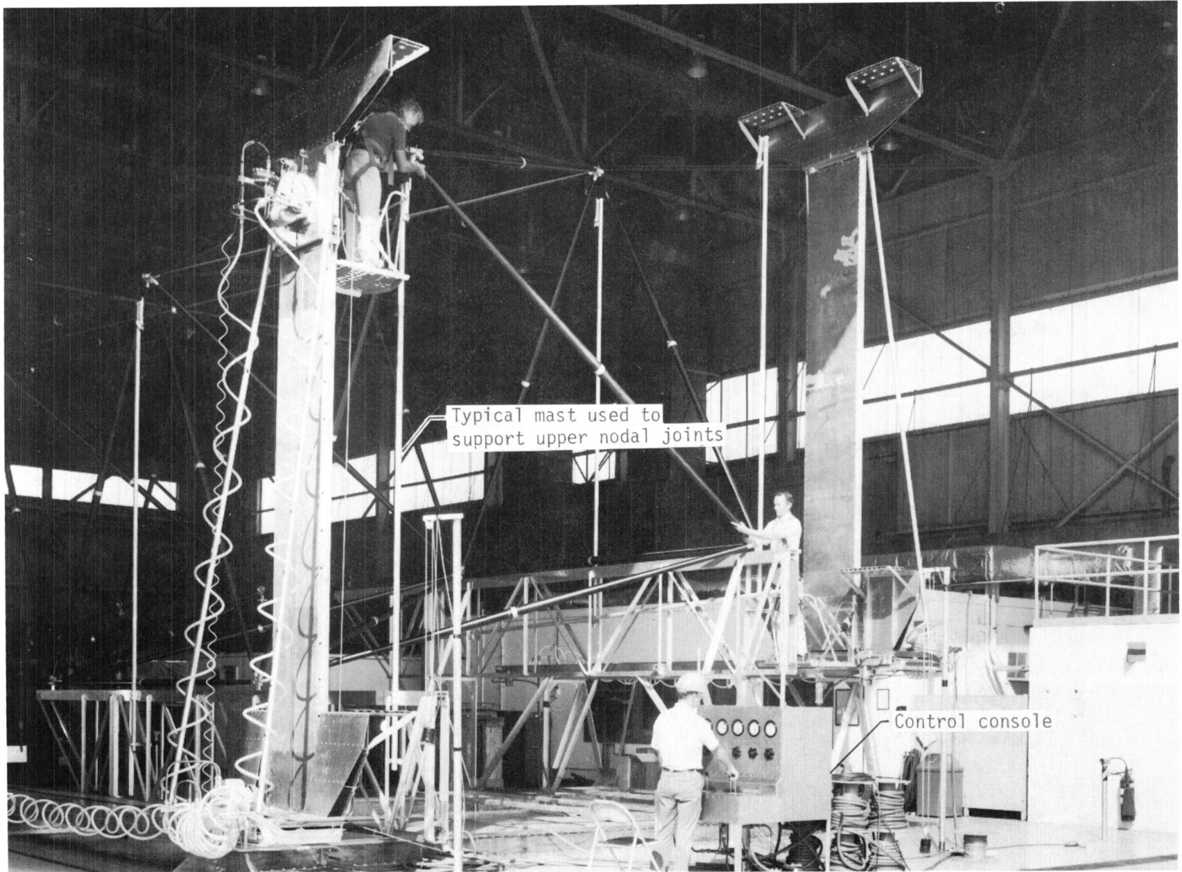
Figure 12.- Setup for 1-g assembly test.
