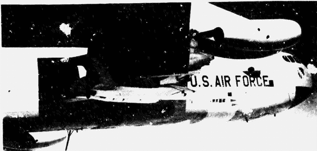
Figure 4. F-15 RPRV on its way to an airborne launch from a B-52 mothership.
