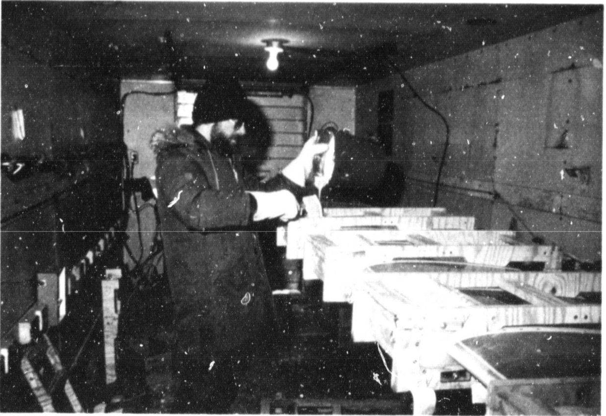
FIGURE 4. Interior of Van Showing Rubber-Mold Boxes Attached to the Rotor Blade.
