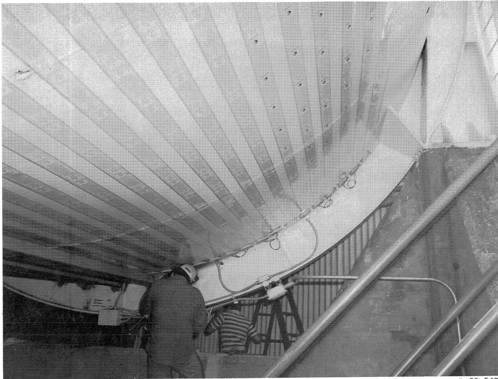
Figure 5.- Photograph of strip-heater installation on outside shell of test chamber.
