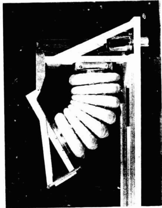
FIGURE IID-5 SHUTTLE/PAYLOAD INTERFACE TUNNEL MODEL - CURVED DEPLOYMENT
