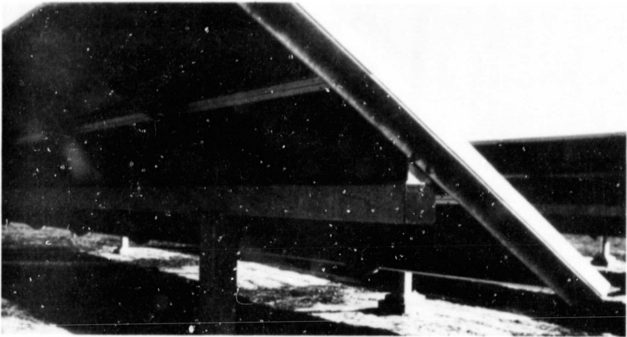
Figure 6. Closeup of PL-120 Mounting Structure
