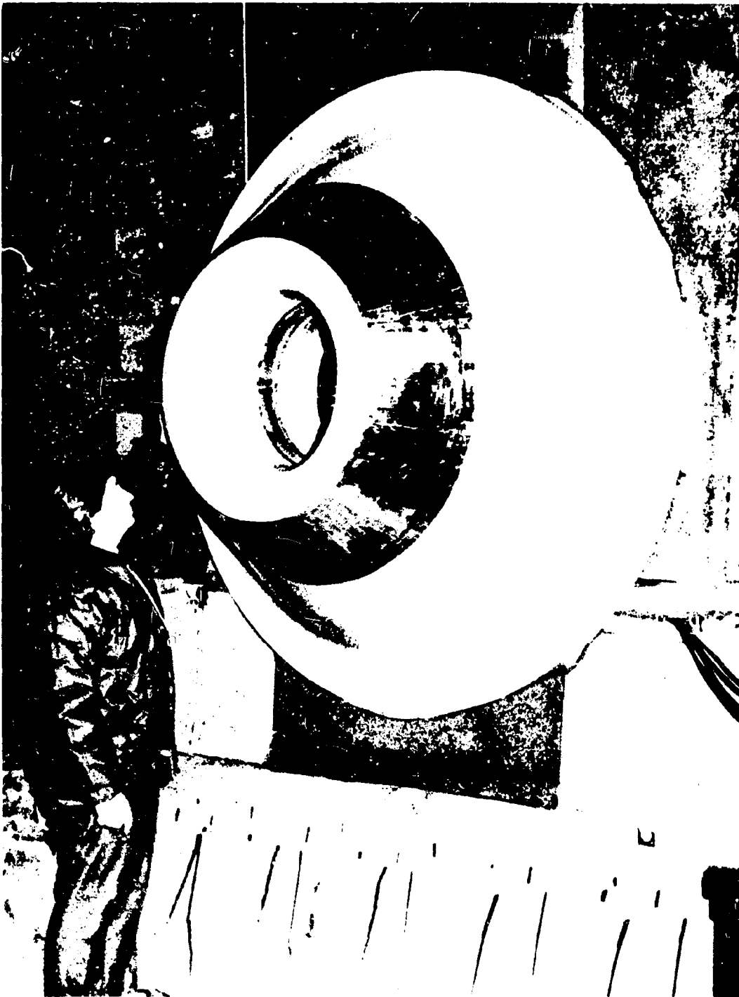
Figure 2. Fan Reverse Cone Inlet Installed.
