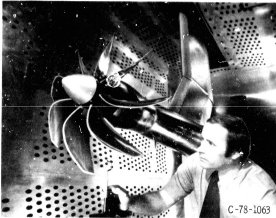
Figure 1. - SR-3 propeller in 8 by 6 foot wind tunnel.
