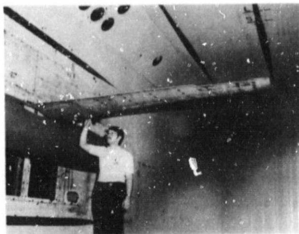
Fig. 30.- Photograph of the fourth model high-aspect-ratio planform (elastic) mounted in TDT.
